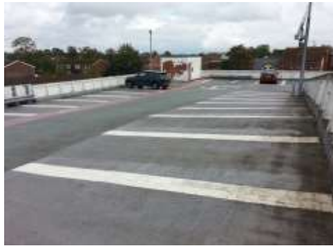
View of old deck.
